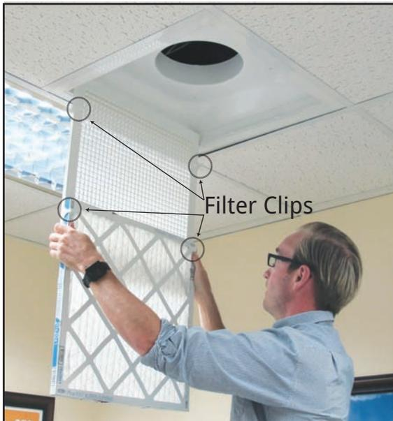
Slide 1" thick filter onto eggcrate face, sliding through filter clips...
