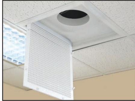
Eggcrate face will hang down on hinges. You can lift off and remove face for cleaning. If inserting or replacing filter leave hanging.
