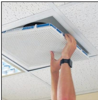
Lift face up and close. Secure by turning the two plastic screw heads with a coin or screw driver.
