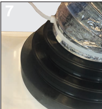
7 Place flexible duct onto reducer and secure with duct strap
