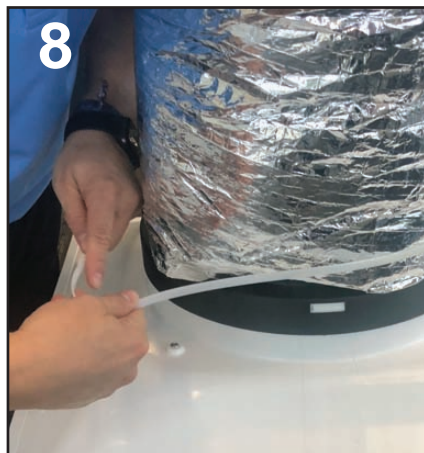
8 Use second duct strap to secure insulation
